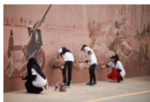
Figure 59. Mural restoration at MS Garrison Underpass, Lahore, 2016. (Source: http://sac.artistan.pk/?portfolio=renovation-of-ms-garrison-underpass-lahore ).
